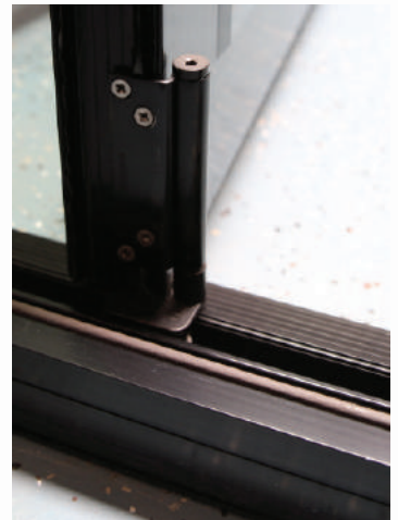
Hinge and door track at sill
